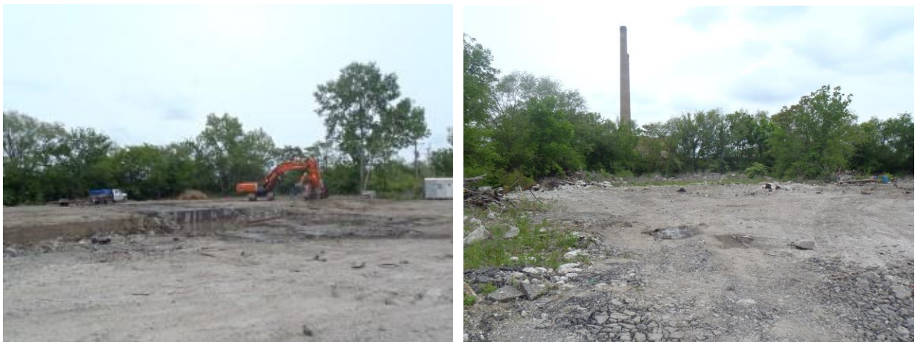
Patriot Tire Shredders site after removal (May 2020)
